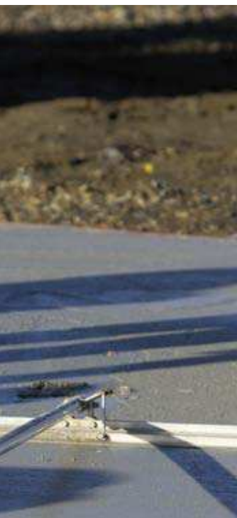
FIGURE 8 Power floating.
