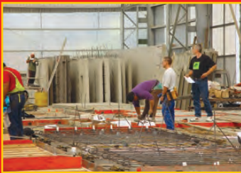
Preparation and production of custom made tilt slab panels
