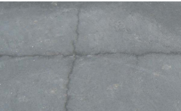
Settlement cracking
